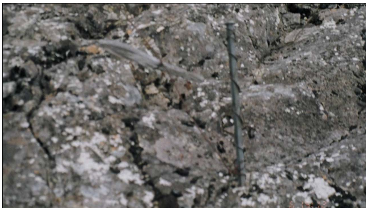
Photo 50- 6: Spike, wire, and wood-splint tensioner for guy wire (center), Knoll site. June 2005.
