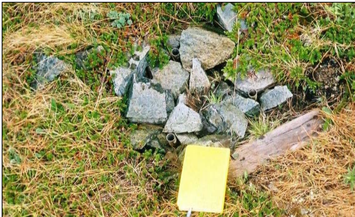
Photo 50- 7: Antenna base on Entrance Point. Three anchors for guy wires were located in triangle array. June 2005.
