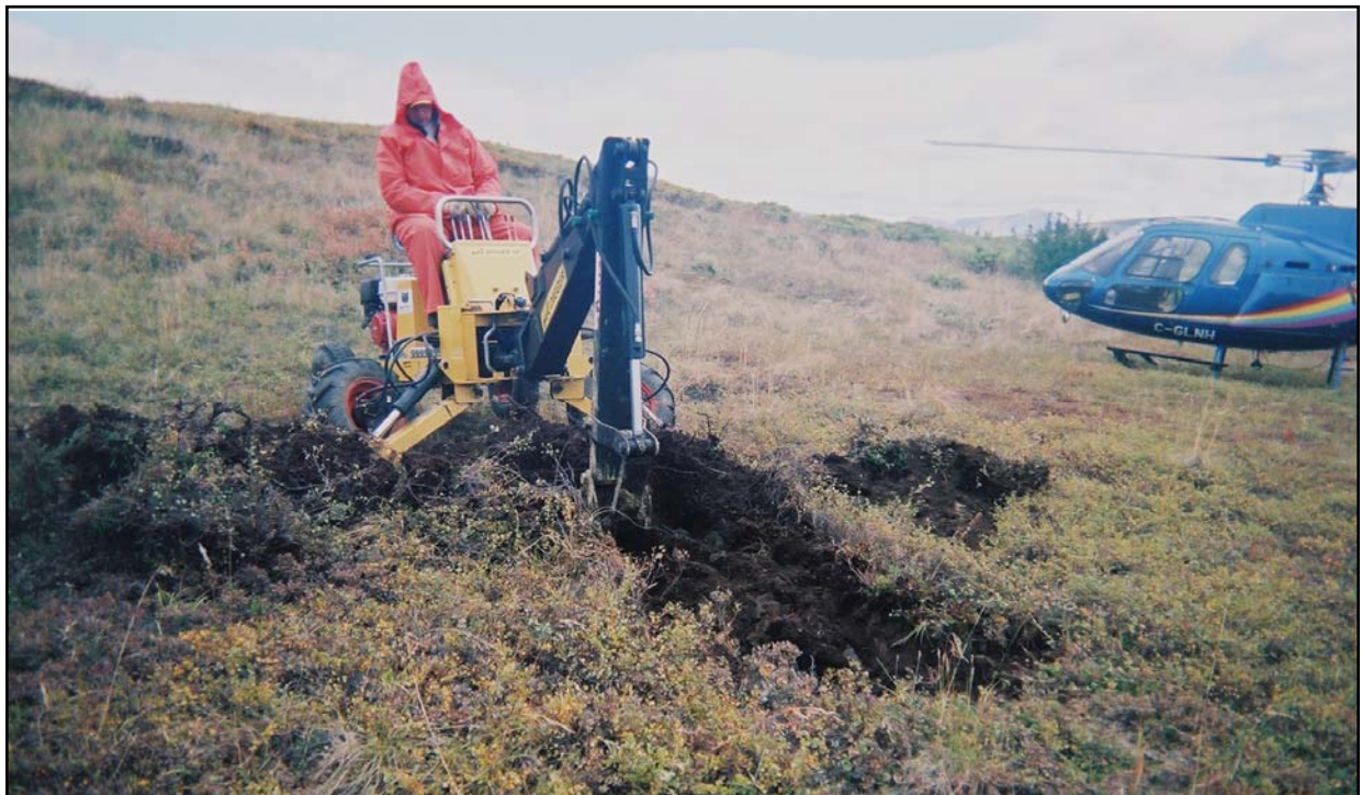
PHOTO 22-26: Excavation of geotechnical assay pit dug with a helicopter-slung excavator. September 2004.
