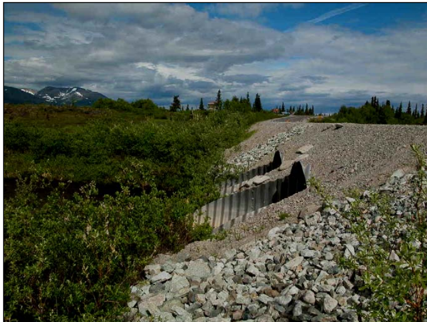
PHOTO 4: GS-20 Roadhouse Creek. Cross-section view of 8-foot culverts to convey flow under road, June 19, 2004.
